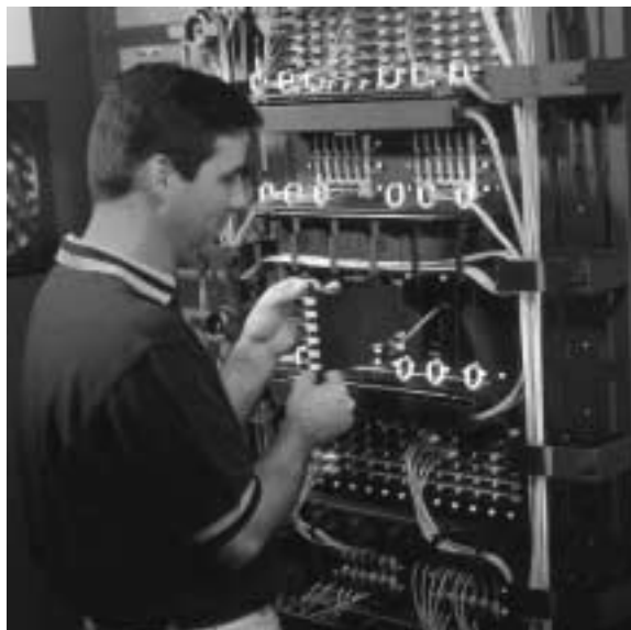
Installation | Photo LAN181A
