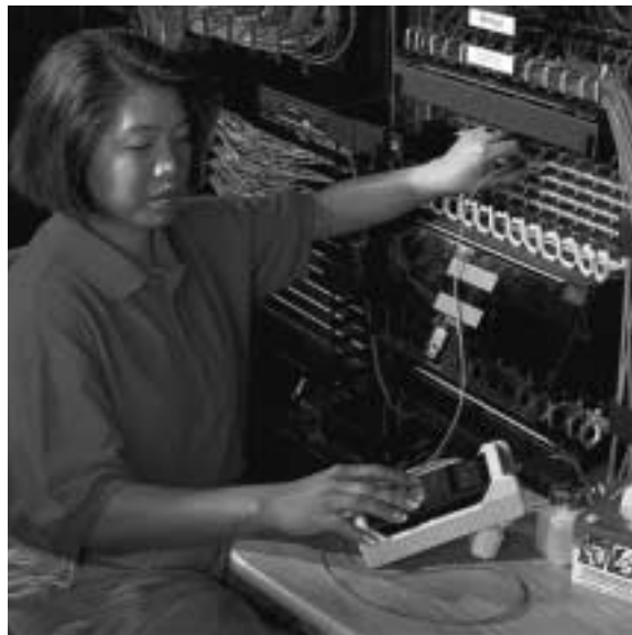
Cable Installation and Testing | Photo LAN79
