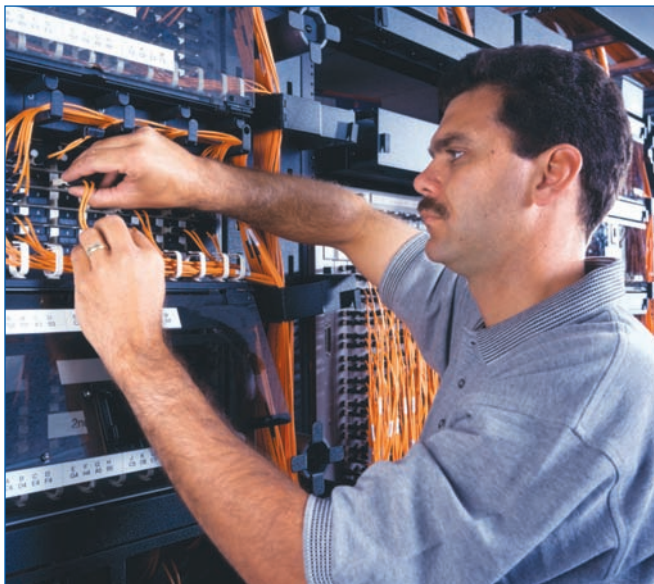
Installation of LANscape Solutions Closet Connector Housings | Photo LAN62
